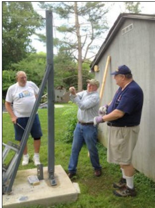
After the tower was lowered, the mast was released and the cable wires were inspected and tested. The brake was clicking, but the rotor would not turn in either direction, emitting a slight hum when the controls were pressed.
